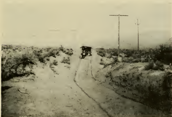
Volcanic ash, which forms the soil of the lower Yakima River country in Washington, may be great for raising crops but, being almost gritless like flour, is a very unsatisfactory material for roads. Great clouds of floating dust hover for hours over the country after the passage of a motor car during dry weather
